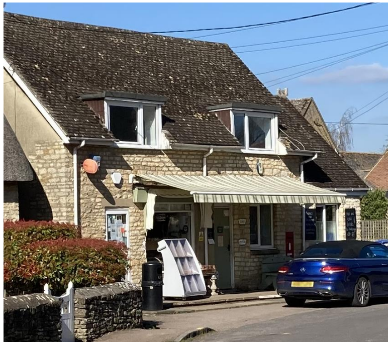
Figure 13 - Weston Pantry Front Elevation Photo
