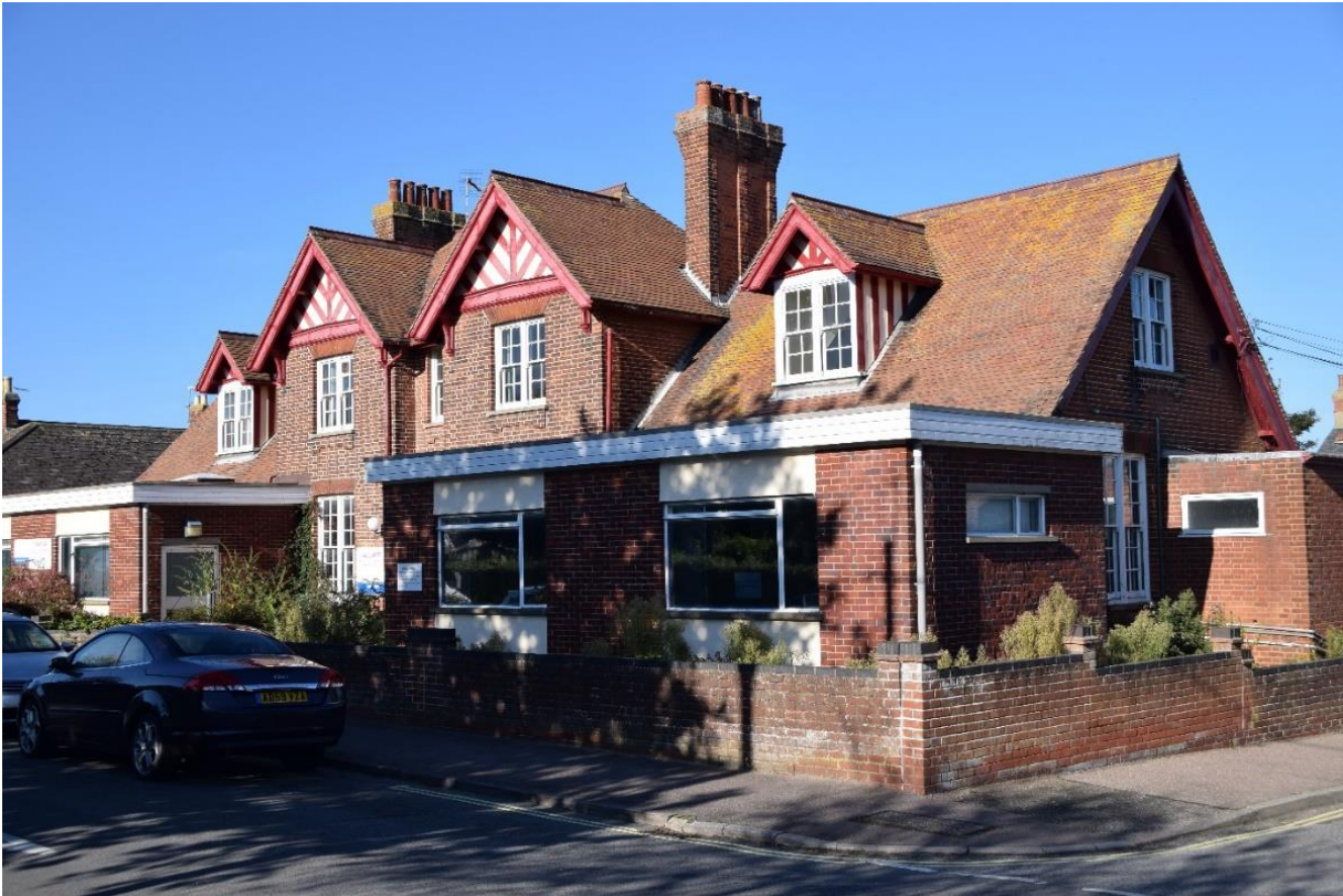
Figure 5 Existing building. Photograph by Rod Tassamini, October 2018.
