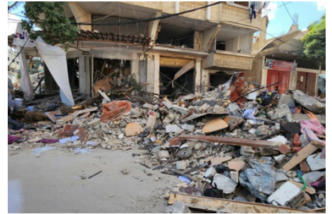
A pile of rubble remains where a building once stood. 18.10.23 © ICRC
